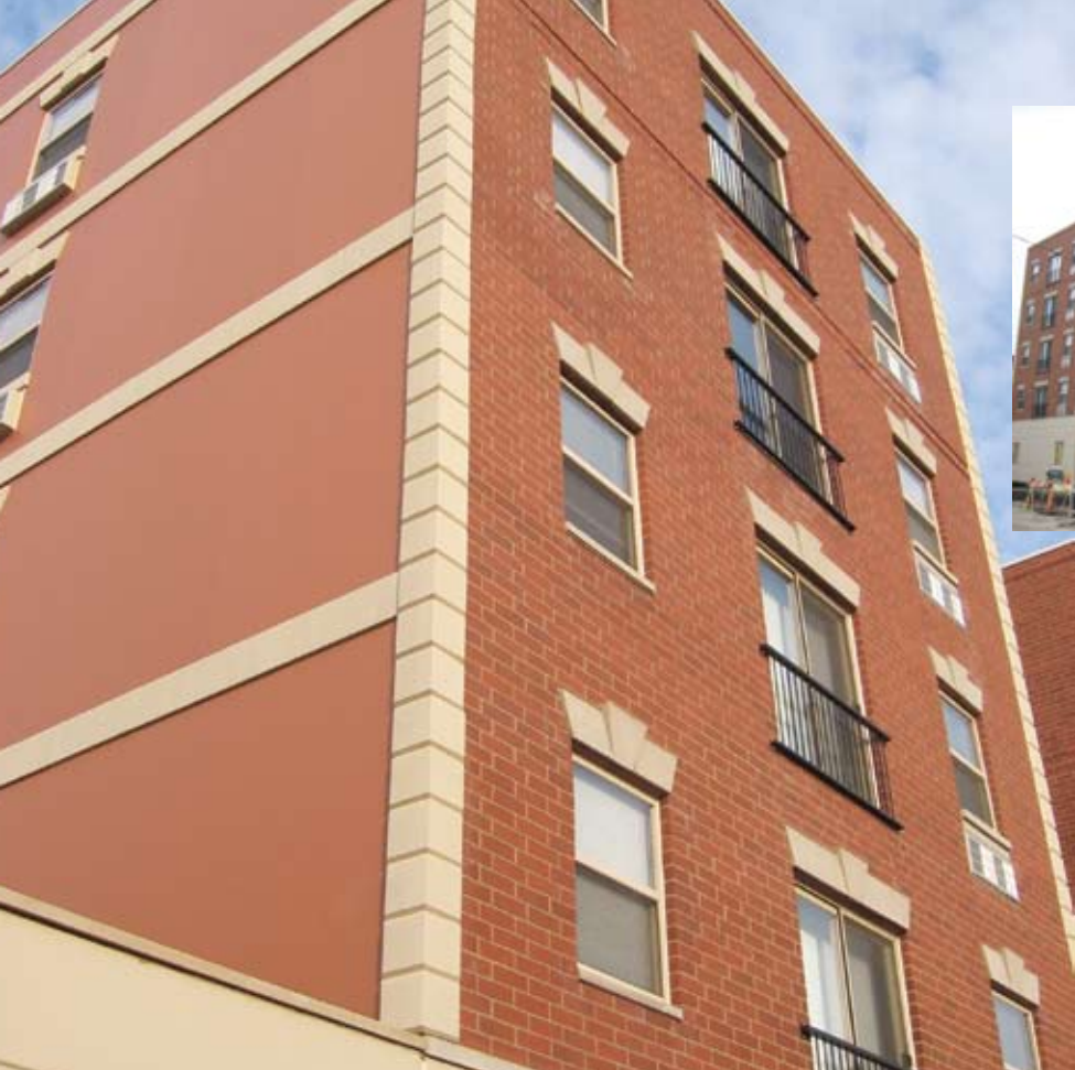
The G&A Residences at Spaulding use Dukane Precast's 8-inch double walls for the exterior walls and 10-inch double walls for flooring, providing high insulation, soundproofing and fire resistance. Photos: Dukane Precast Inc.
