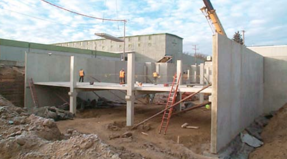
Using a new two-story foundation wall from Molin Concrete Products Co. for an apartment building at 808 Berry Place in St. Paul, Minn., designers value-engineered the foundation from masonry to precast, worked through the coldest winter months at a lower cost, and reduced construction time by eight weeks. Photos: Molin Concrete Products Co.
