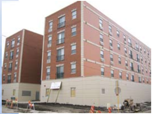
The G&A Residences at Spaulding on Chicago's Northwest Side use Dukane Precast's double-wall system. The panels on the sides and rear of the building have cast-in brick reveals that are painted.
